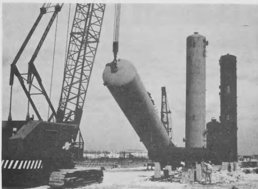
AT THE Barcadera industrial site, a heavy-duty crane positions a first-stage absorption tower. The big tower is one of many process units that will make up the Antilles Chemical Company plant. It weighs nearly forty-three tons and stands nearly sixty feet in the air.
